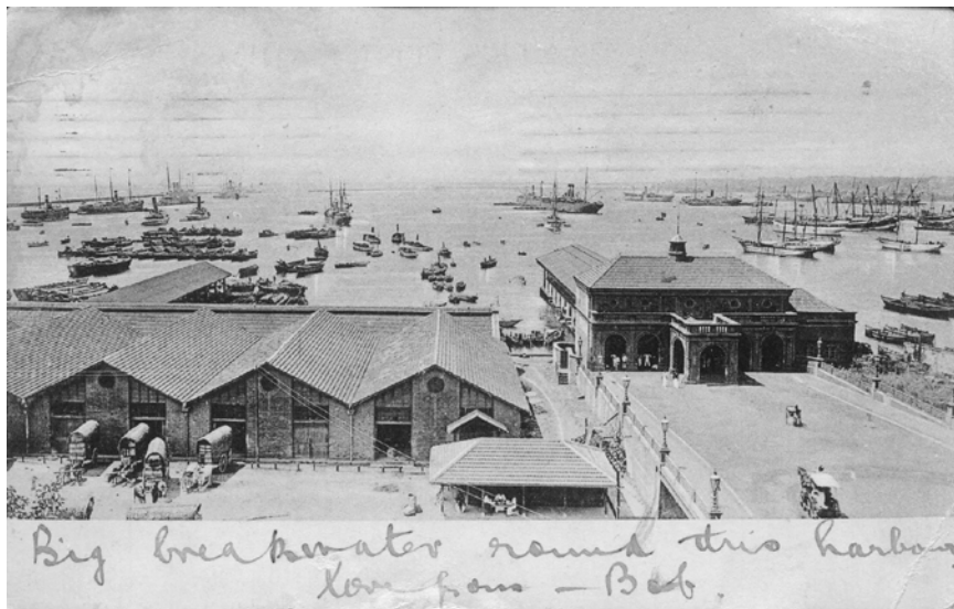
Colombo Harbour and Jetty
